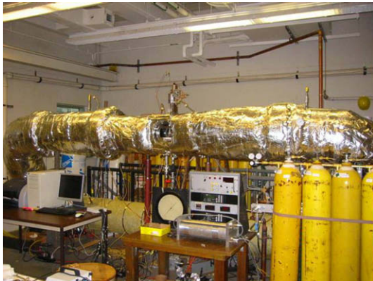
Fig. 3. Photograph of the heat transfer tunnel with insulation.
